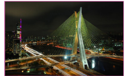
Ponte Estaiada Octavio Frias de Oliveira http://www.skyscrapercity.com/member.php?u=449572
